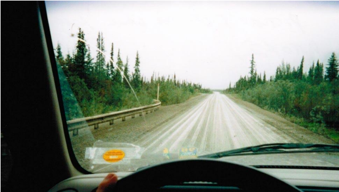
This is the haul road and as you can see from the photo it can get very slick and greasy when it rains.
