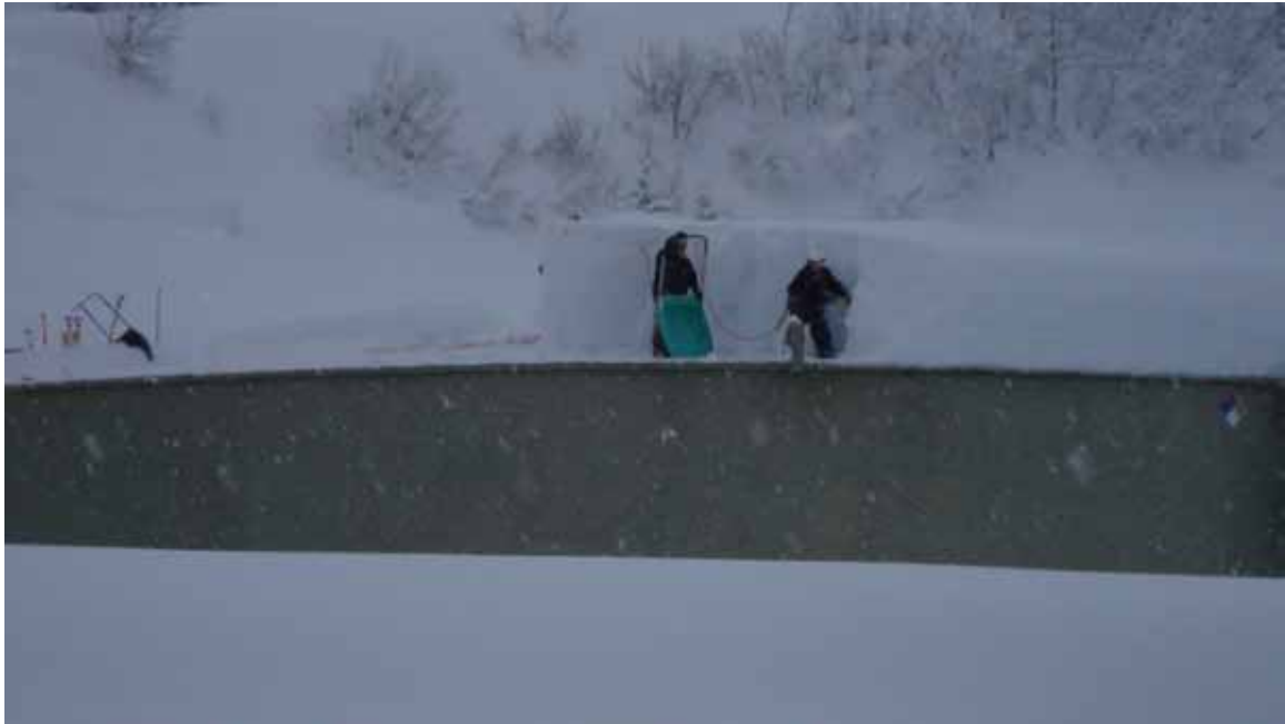
Shoveling snow off of a tank top
